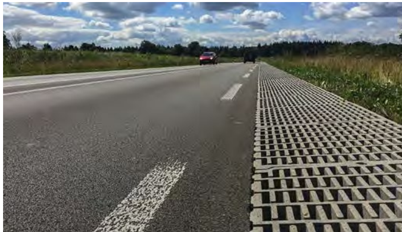
Figure 4-10 – Horizontal Lattice Structure Example
